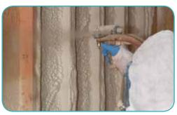
Benefits: CertaSpray Closed Cell Foam provides thermal insulation for the interior or exterior of the building and reduces air infiltration through the building envelope.
