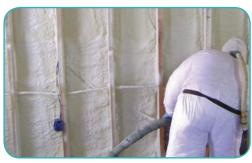
Benefits: CertaSpray Extreme Winter Closed Cell Foam provides thermal insulation for the interior of homes and commercial buildings, and reduces air infiltration through the building envelope.
