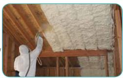
Applications: The open cell low density foam can be spray-applied into open wall cavities, perimeter joists, cathedral ceilings, garage ceilings, attics and crawlspaces. Product can be installed up to 12" thick in ceilings and walls when covered with a code-approved 15-minute thermal barrier. Product is meant for interior applications. Product must be finished according to local code, and must be applied by a qualified applicator.
