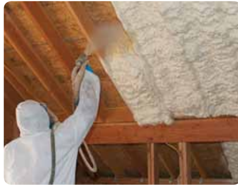
Spray Foam Insulation
