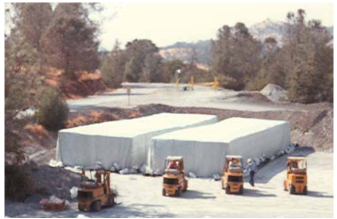
Construction Site Covers
