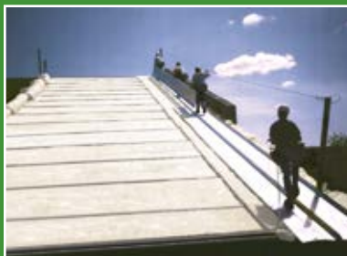
Install JM Formaldehyde-free™ fiber glass insulation between and over purlins.
