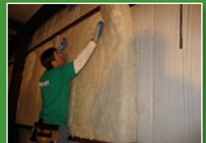
Insulation is cut to fit the full space and impaled on the Fast-R™ hangers.
