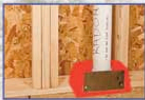
Seal radon gas entry routes.
