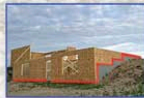
Prevent dust and moisture entry through plate lines.
