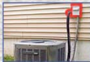
Seal air conditioning penetrations.
