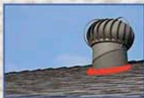
Close leaky gaps in attics and roofs.
