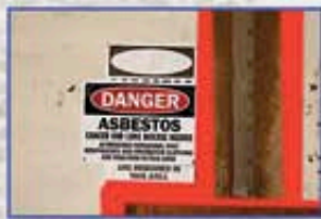
Positive air sealing in asbestos removal areas.
