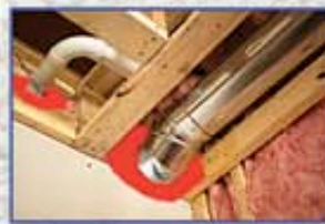
Seal utility penetrations.
